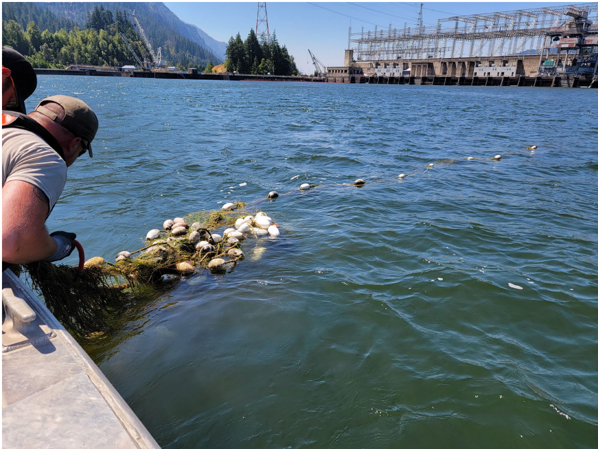
Figure 2. Removal of large gill net in PH1 Forebay BRZ
